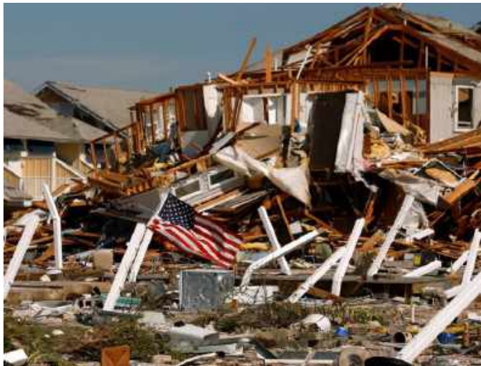
Hurricane Michael damage in Tallahassee, Florida
